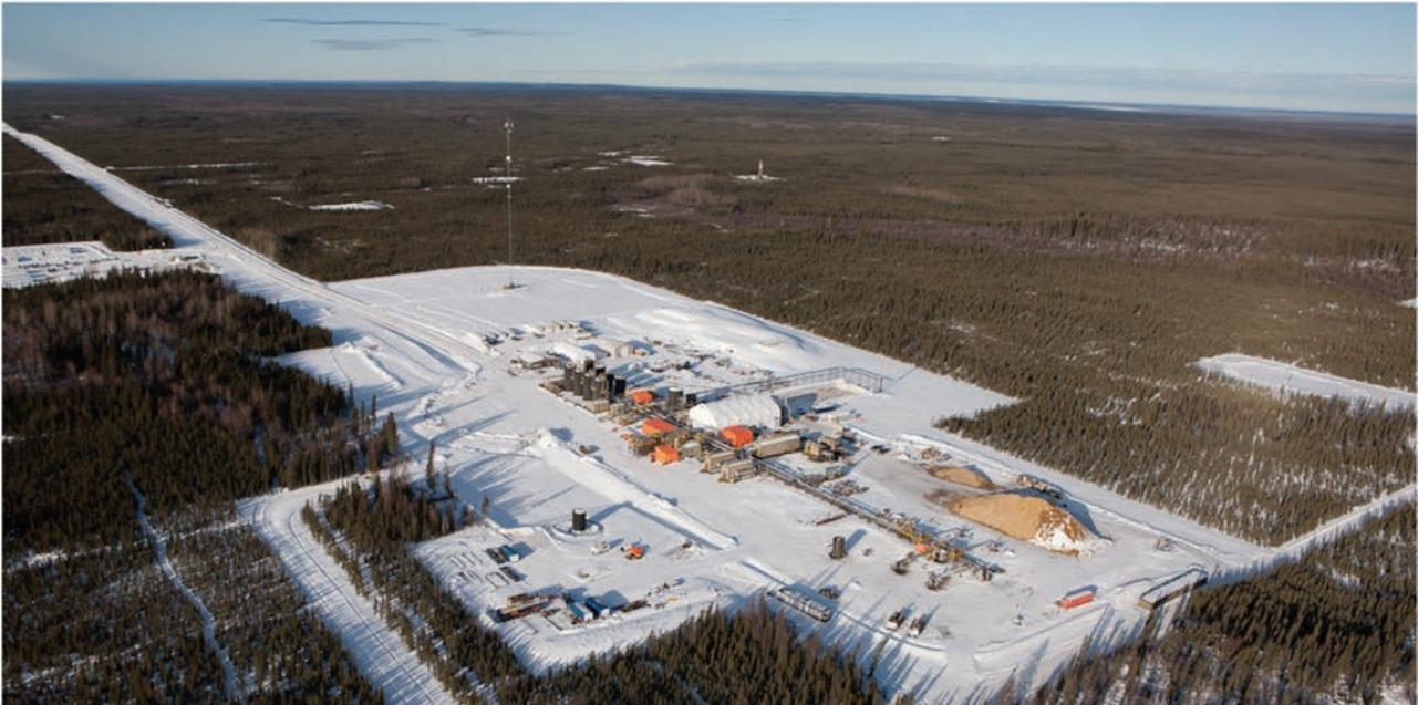
This clearing was used for a pilot project testing bitumen production from the Grosmont Formation by a joint venture formed by Laricina Energy and Osum Oil Sands. They needed to build a road to the remote location in north central Alberta where they used various heating methods to produce the heavy crude from a carbonate formation.
